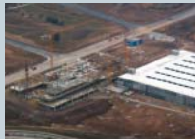
In Neckarsulm the new affiliate company is built at Bechtle-Platz 1
