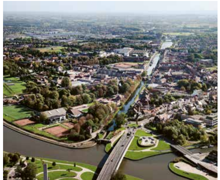
Upgrading the Bossuit-Kortrijk Canal
