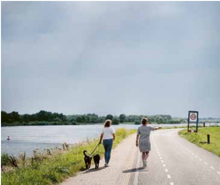
Flood protection between Tiel and Waardenburg
