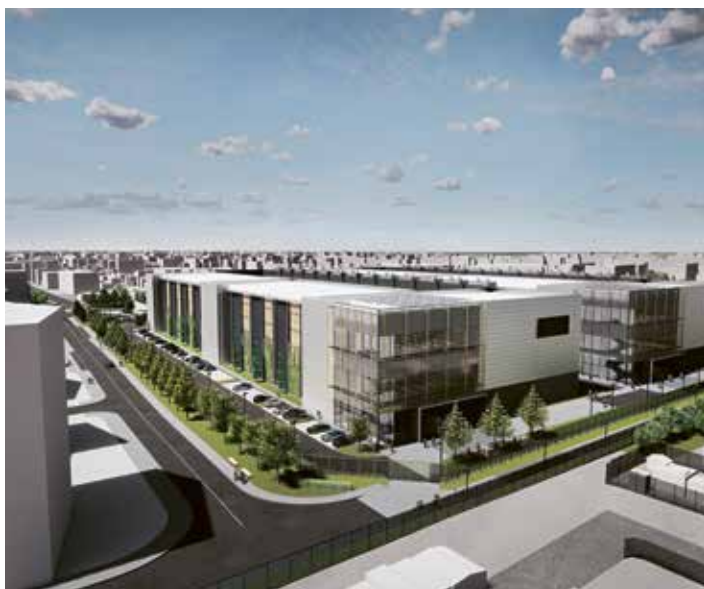
Data centre in the outskirts of London
