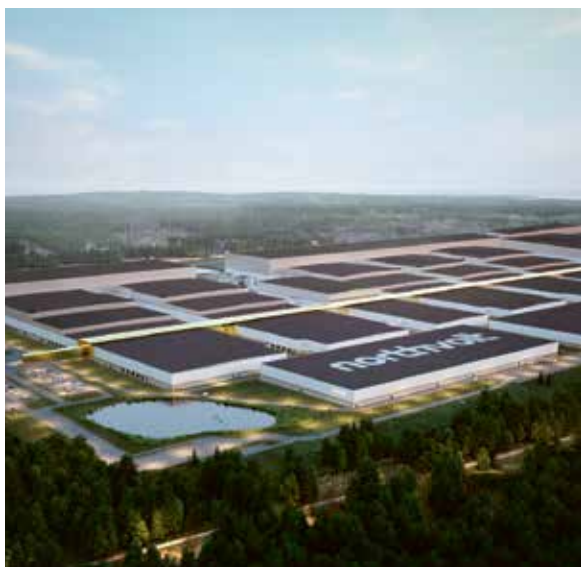
Battery manufacturing plant for Northvolt
