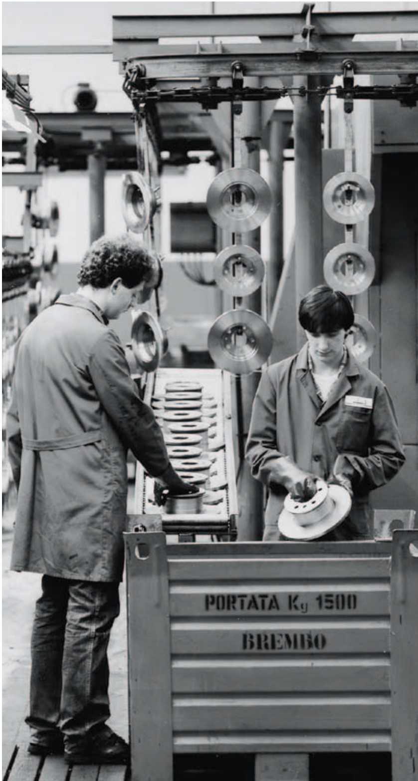
Production line for car discs at the plant in San Giovanni Bianco (Bergamo).
