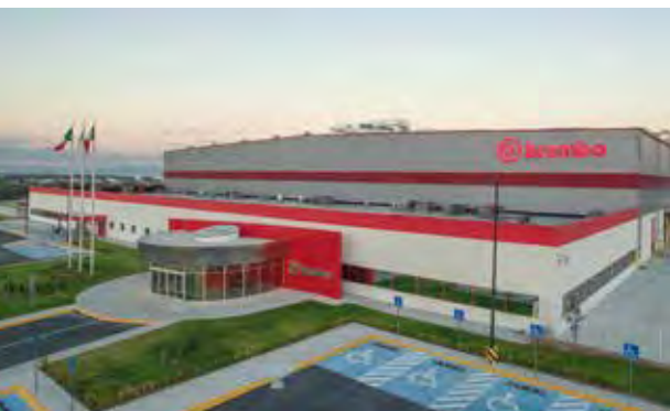
The new integrated plant for the production of aluminium calipers in Escobedo, Mexico.
