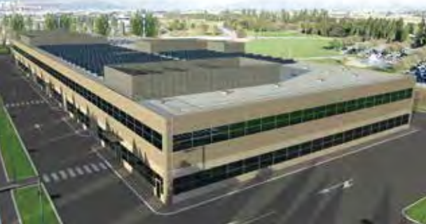
The new facilities of the Testing Department in Stezzano (Italy).
