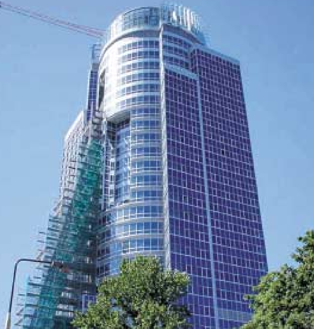
With 32 floors above ground and five below, the Polish Telecom headquarters in Warsaw is the tallest building designed by a Polish architect. The 1500 steel, aluminum or wooden doors are linked into a three-level masterkey locking system based on ABLOY DISKLOCK PRO technology and combining ABLOY mechanical and electromechanical cylinders and FUNXION door hardware.
